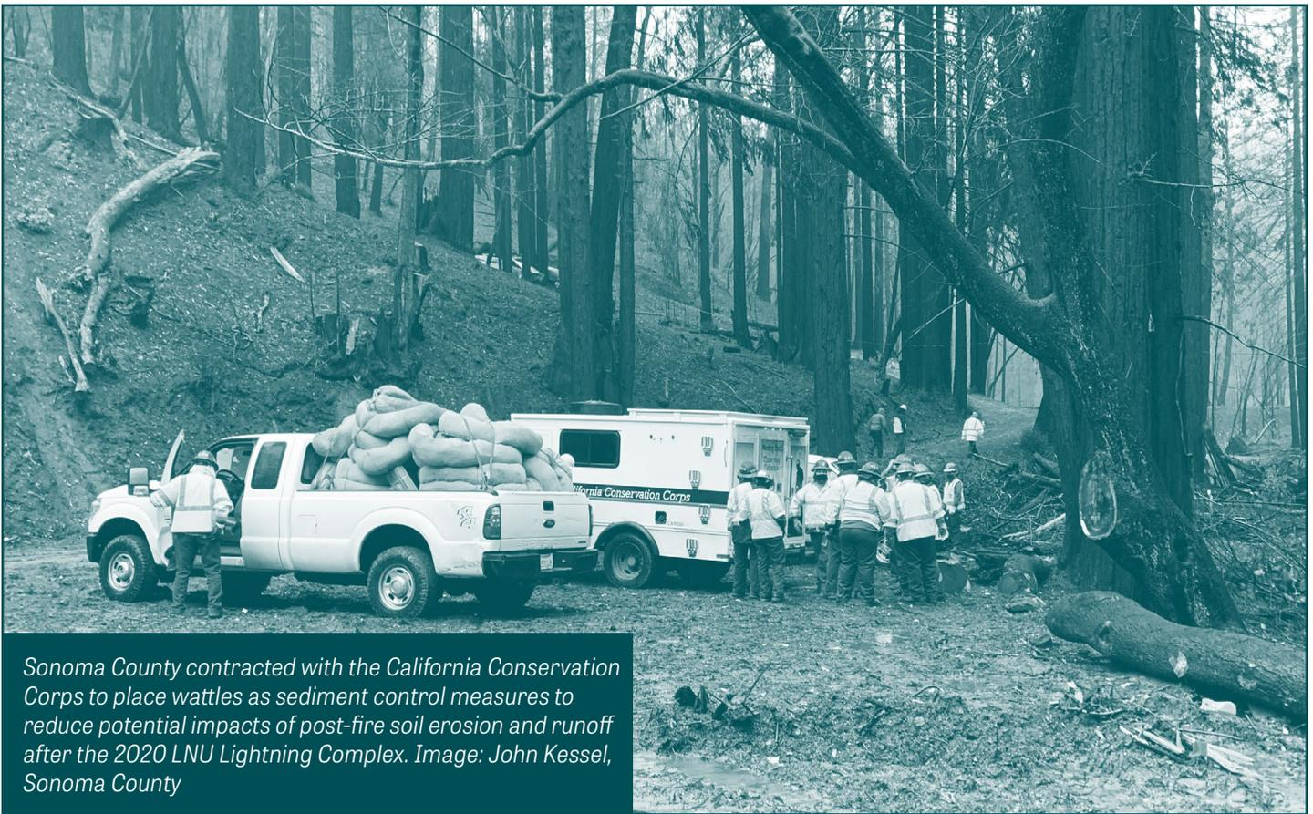
*Sonoma County contracted with the California Conservation Corps to place wattles as sediment control measures to reduce potential impacts of post-fire soil erosion and runoff after the 2020 LNU Lightning Complex. Image: John Kessel, Sonoma County*
